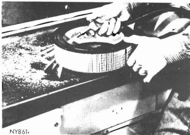
Fig. 4 - Cleaning air filter
